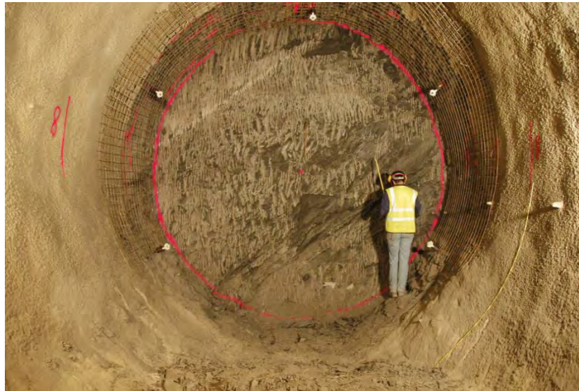
Figure 4.38. View of FE tunnel face from the FE niche showing beddings dipping 45° (Vietor, 2012).
